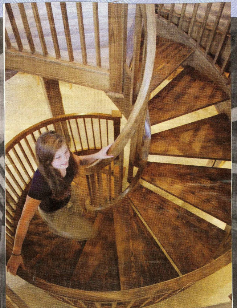
It took master builder Phil Lafreniere about three months to build the staircase.
